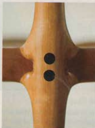
The Butterfly Joint has curved edges and transfers a sitter's weight into a chair's vertical grain.
